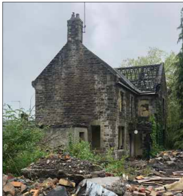
North east elevation from within the site
