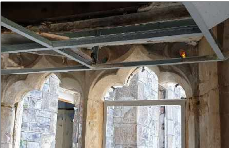
WF7 - First Floor. Tear drop elements in direct glazed coloured glass, to be retained.
