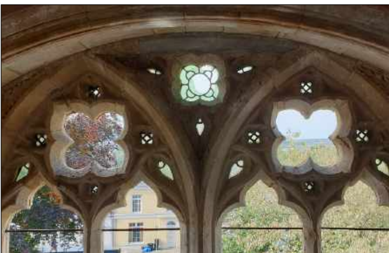
WS1 - Second Floor. Clear glazed leaded lights, to be retained or, where necessary, repaired and replaced.
