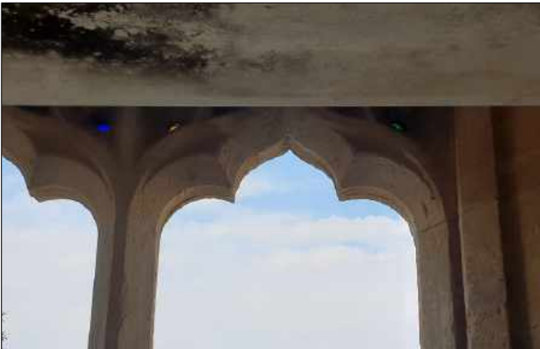
WF6, First Floor. Tear drop elements in direct glazed coloured glass, to be retained
