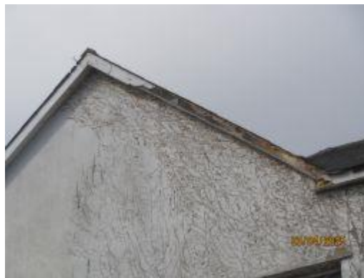
Eastern elevation – PRFs – missing bargeboards with gaps providing access to a cavity between a layer of bitumen felt and slate.
