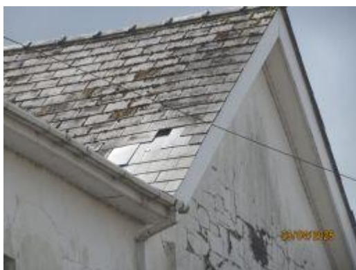
Missing slate providing access to a cavity between a layer of bitumen felt and slate.
