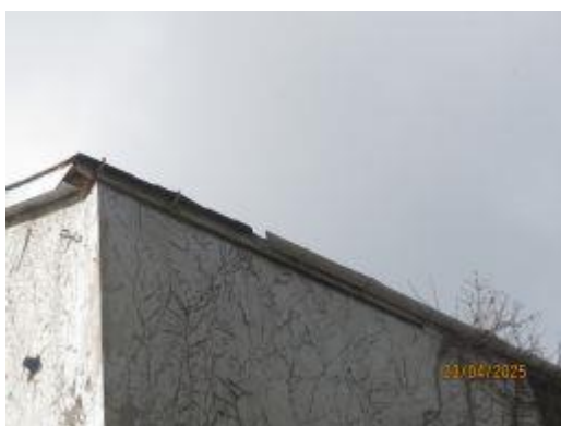
Northern elevation – PRFs – missing bargeboards with gaps providing access to a cavity between a layer of bitumen felt and slate.
