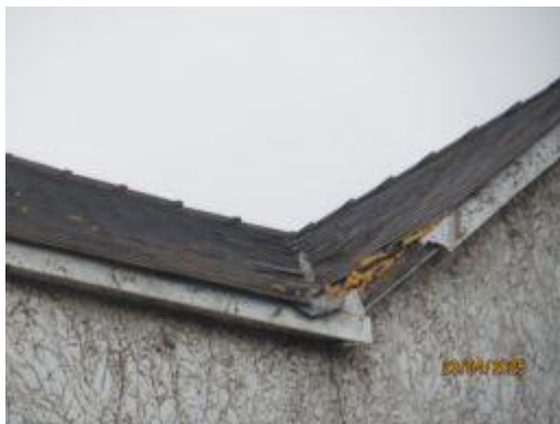
Eastern elevation – PRFs – missing bargeboards with gaps providing access to a cavity between a layer of bitumen felt and slate.
