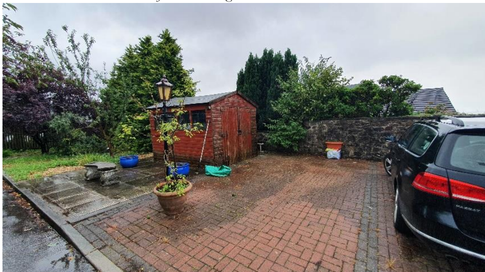
Photo 1: Overview of hard standing.
