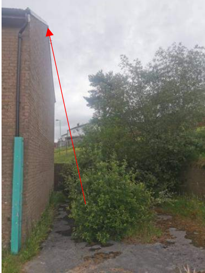
Figure 5- common pipistrelle emergence point (arrowed red)
