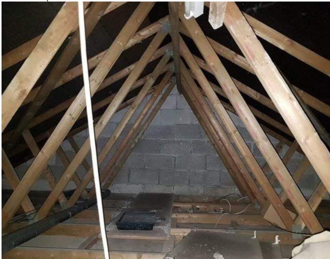
Block 3 roof space
