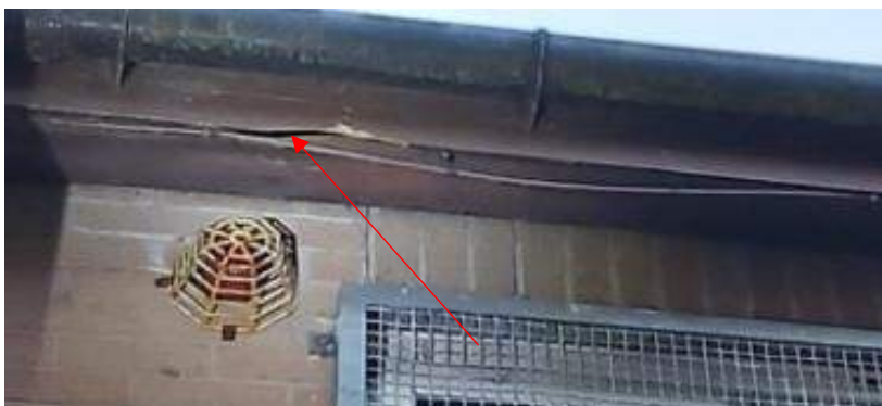
Figure 6- common pipistrelle re-entry point (arrowed red)
