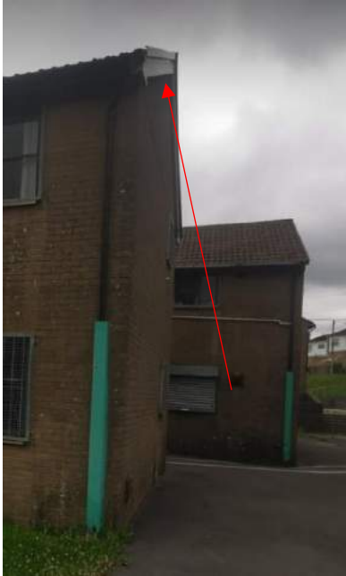
Figure 4- common pipistrelle emergence point (arrowed red)
