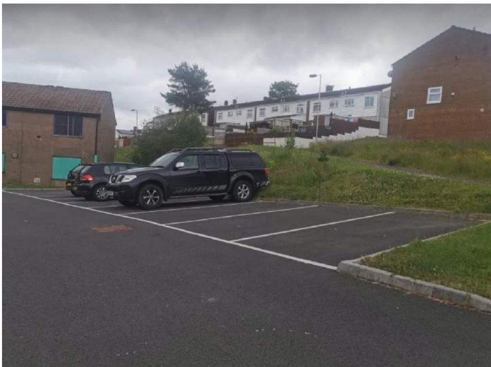
Plate 2- view of rear car park
