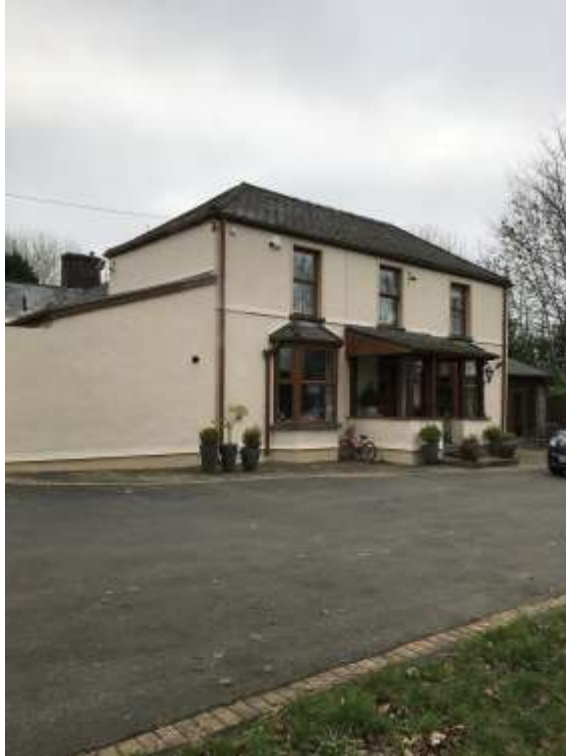
Plate 5- photograph of the north west elevation of the existing house
