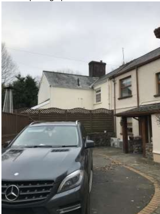
Plate 6- photograph of north east elevation
