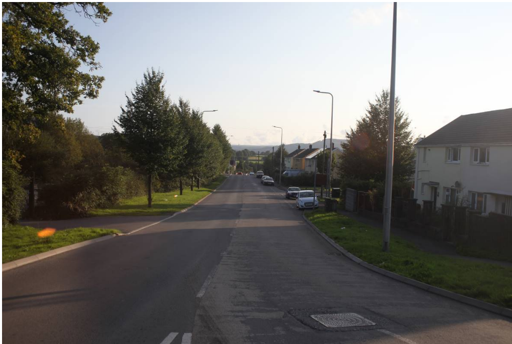
View along Gelligaer Road, site is to the left hand side, after road access to Cath's Farm Shop, behind lime trees in verge.
