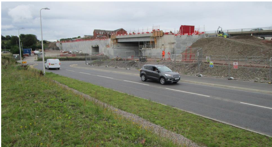
Cheltenham Avenue in July 2023. The eastbound carriageway of the A465 is under construction, obscuring much of the MMA yard.
