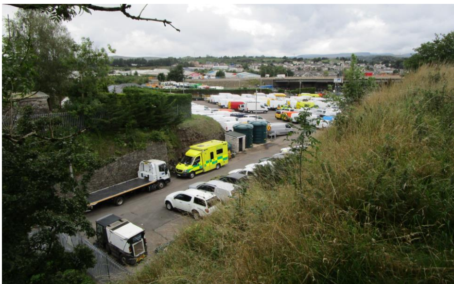
View of MMA yard (2023) looking north from rock cutting showing the A465(T) flyover
