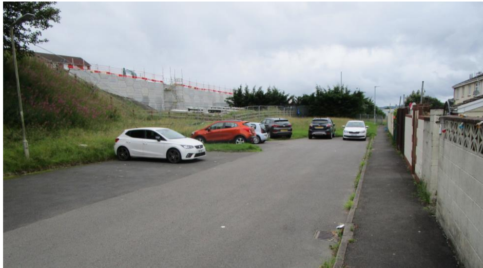
View (2023) along the southernmost access road into the Hafod (R4). The evergreen hedge (centre) will remain. The new retaining structure of the A465 eastbound carriageway is visible at centre left
