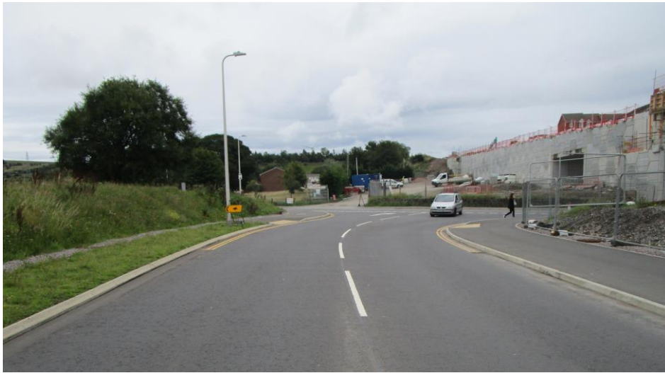
View from realigned Cheltenham Avenue (R6). A465(T) to the right (under construction), existing MMA site in centre, Amenity area to the left of the Cypress hedge
