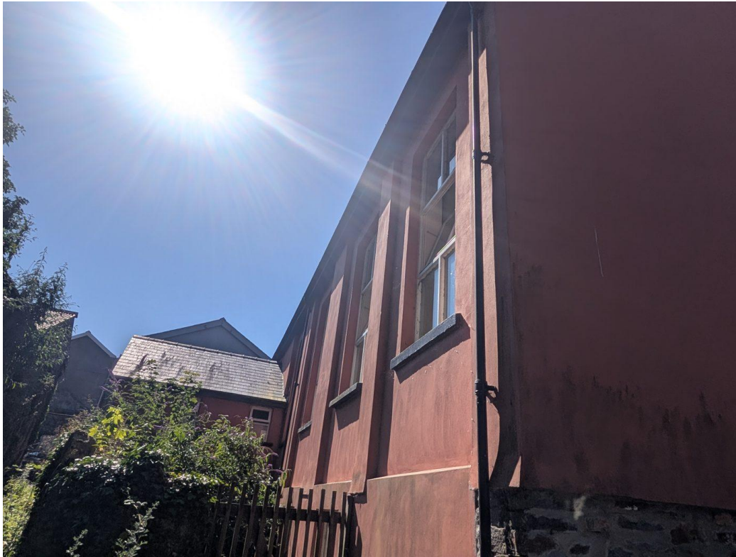
Plate 3 – Rear elevation of the vestry and schoolroom range, showing sound render, cast iron rainwater goods and closely laid slate roof beyond.
