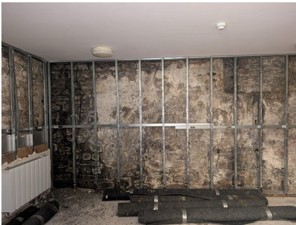
Plate 6 – Basement level, showing exposed coursed rubble stone perimeter wall, new galvanised metal stud framing and intact plasterboard ceiling. No evidence of bats was recorded.
