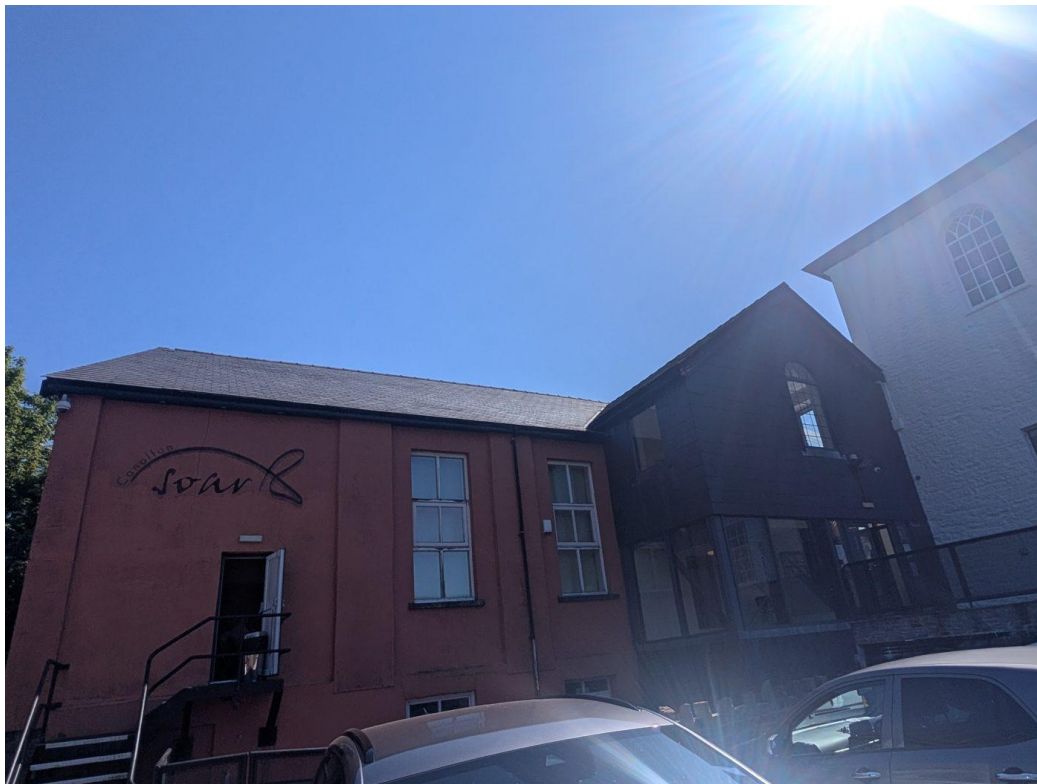
Plate 2 – Vestry and schoolroom range, showing painted render, timber sash windows, boxed painted eaves and natural slate roof in good condition.
