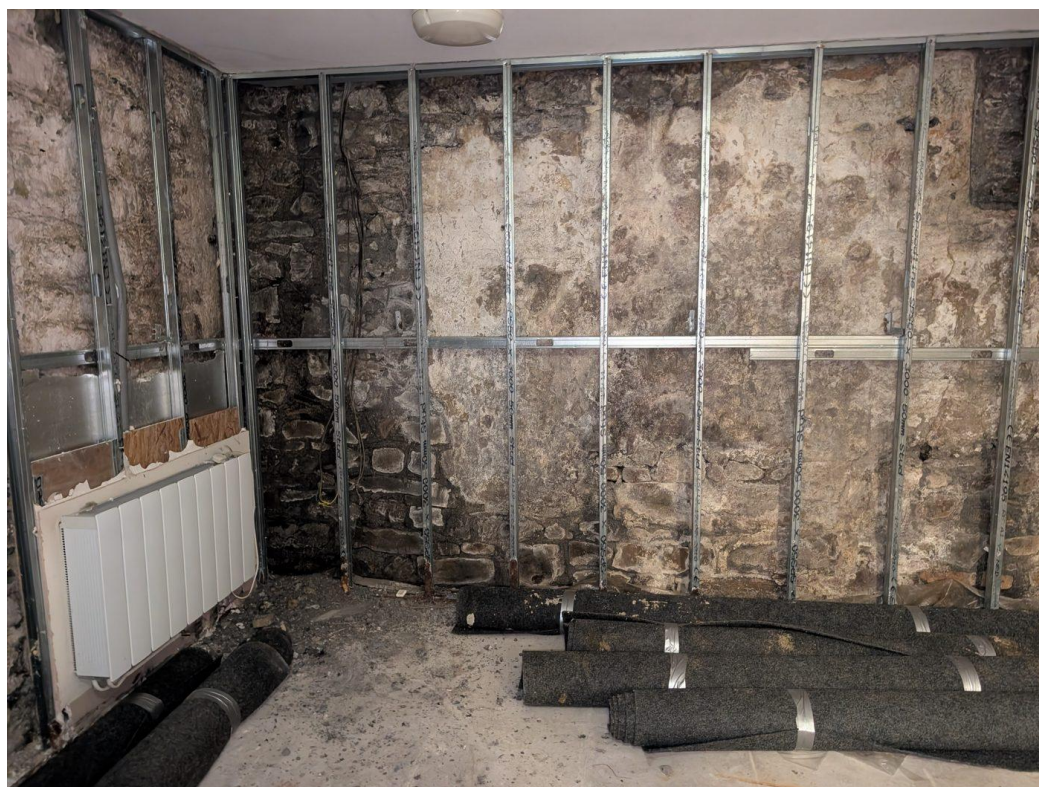
Plate 7 – Basement level, alternative view of the stripped perimeter wall and stud framing prior to re-lining.
