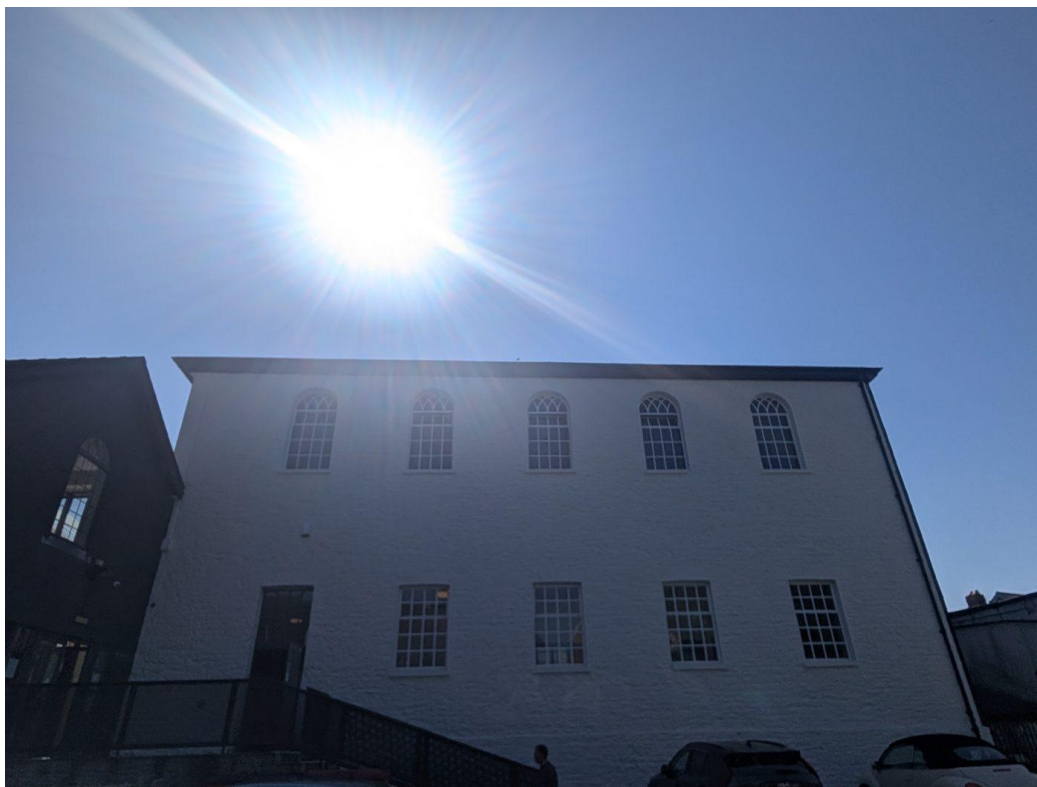
Plate 1 – Chapel elevation, showing painted render, round-arched first floor windows and closely detailed slate roof with no access points for bats at eaves level
