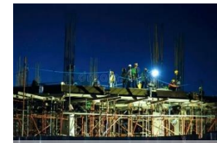
Fig.3.12 – Local task lighting
