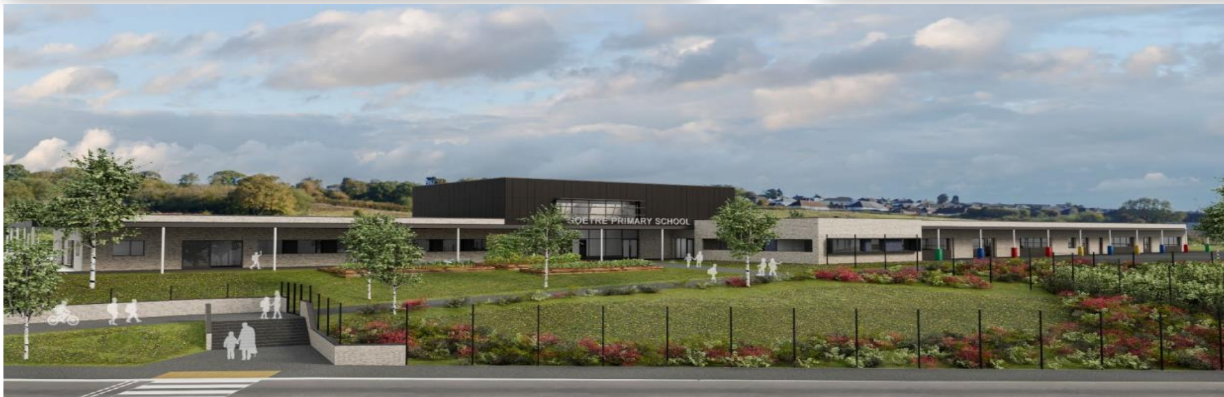
View Of Goitre Primary School from the Southwest off Goitre Lane
