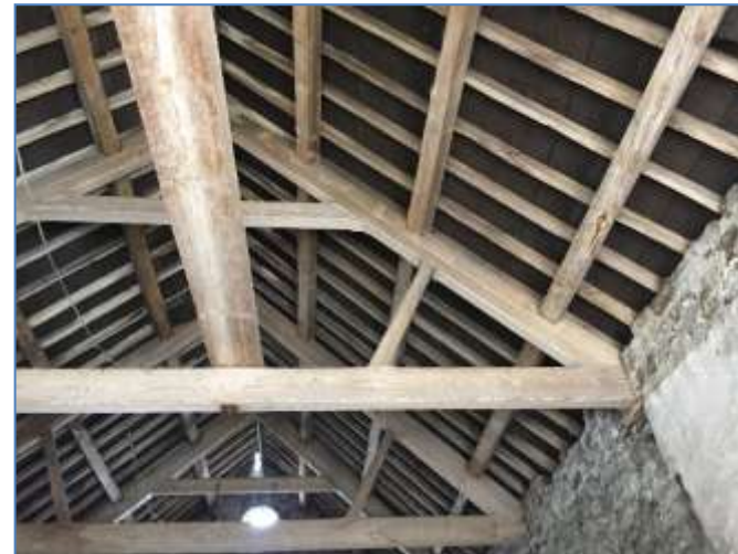
Photograph 12. Building B, western section . The tie and collar beam roof construction.
