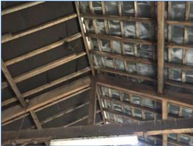
Photograph 29. Building F. The unlined slate tiles on the southern pitch and bitumen felt on the north.
