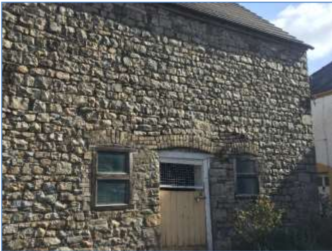
Photograph 3. Building B, eastern section. The rough stonework on the southern elevation.
