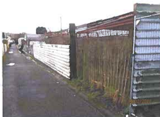
Figure A7.3: The eastern boundary looking south from the northern corner. There are a mixture of materials including Heras fencing, wooden fencing, corrugated sheeting and wire fence.
