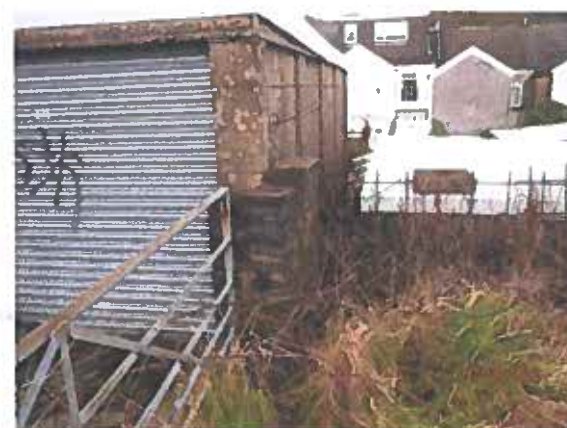
Figure A7.4: The northern boundary taken from the western corner. The garage to the left is a neighbouring property and the white roof (centre-right) belongs to the on-site store/workshop.
