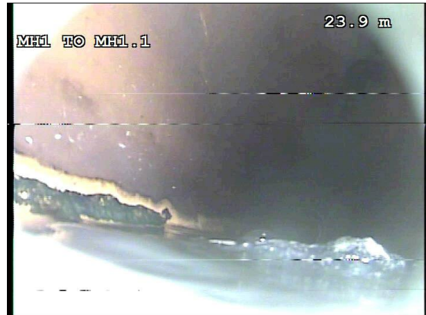
Photo: 60_9a, 00:00:00 23.9m, Water level, 20 % height/diameter
