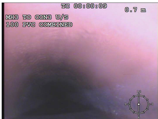
Photo: 45_4a, 00:00:00 0.7m, Water level, 50 % height/diameter
