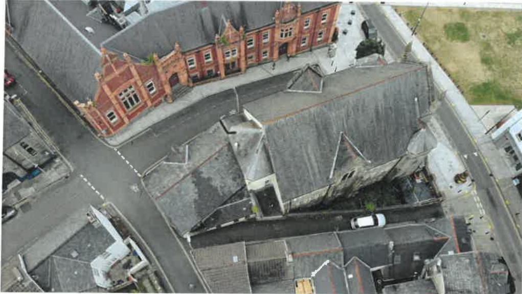
Overview of the roof.
