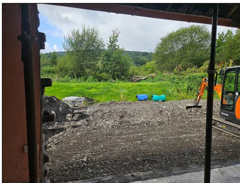
Figure 9: The view from inside the building showing some of the surrounding vegetation and stone piles
