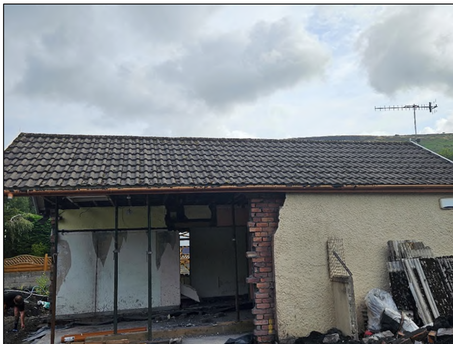
Figure 5: The building from the South side.
