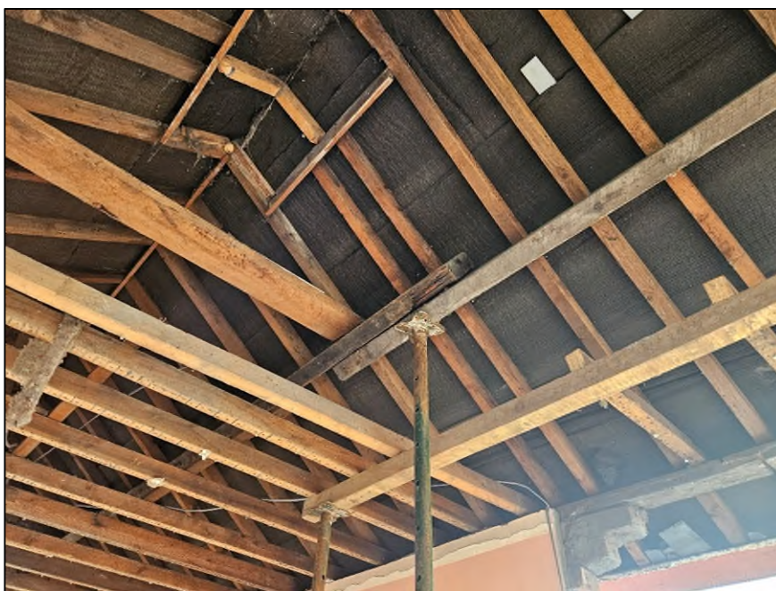
Figure 8: The roof and attic space
