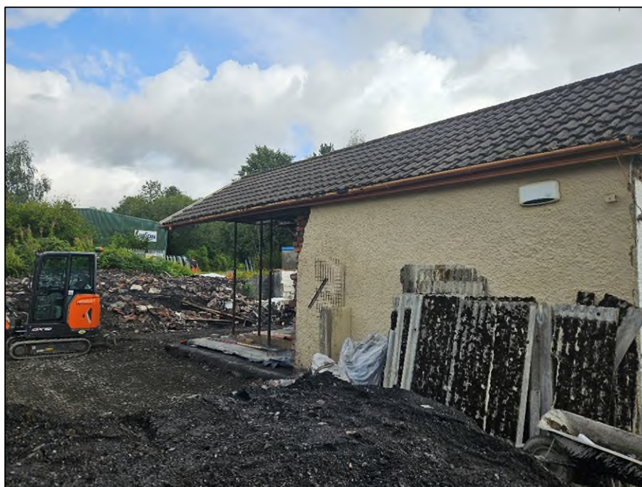
Figure 6: A view of the South side of the building with the piles of stone
