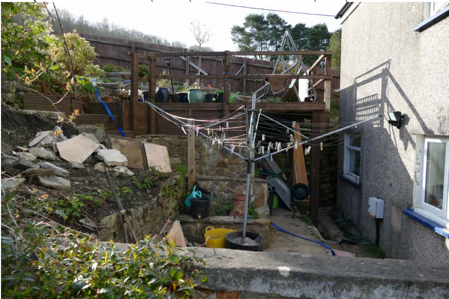
General View Into No.1 Showing Patios and Raised Decking
