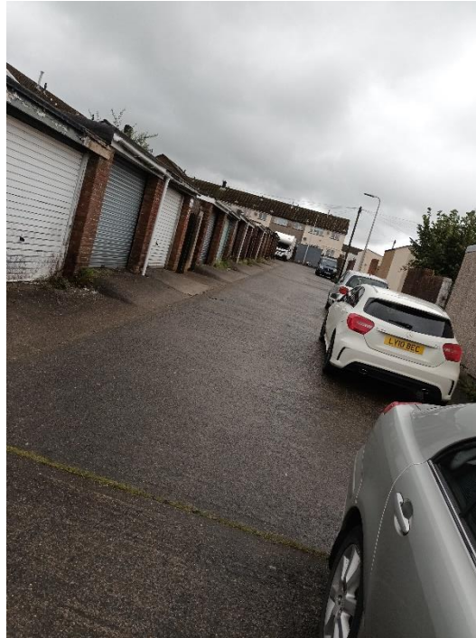
Plate 1-Lighting columns on the front elevation of the garages.
