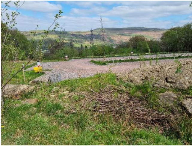
Figure 15 – View south across new car park area.
