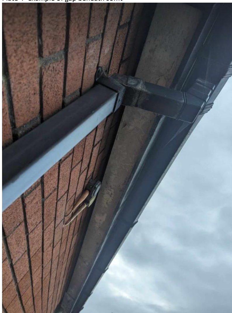
Plate 4- example of gap beneath soffit
