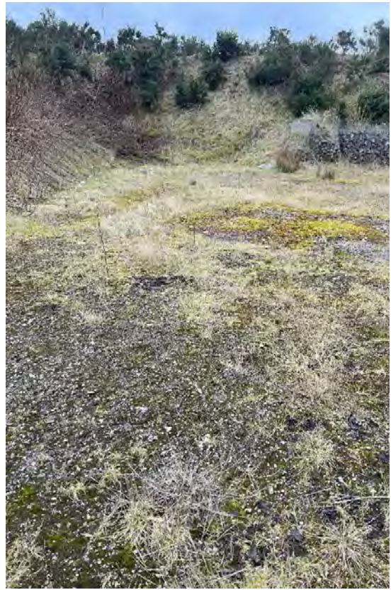
Image EDP A3.2: Ephemeral/short perennial vegetation encroaching into the centre of the Site across areas of hard standing.
