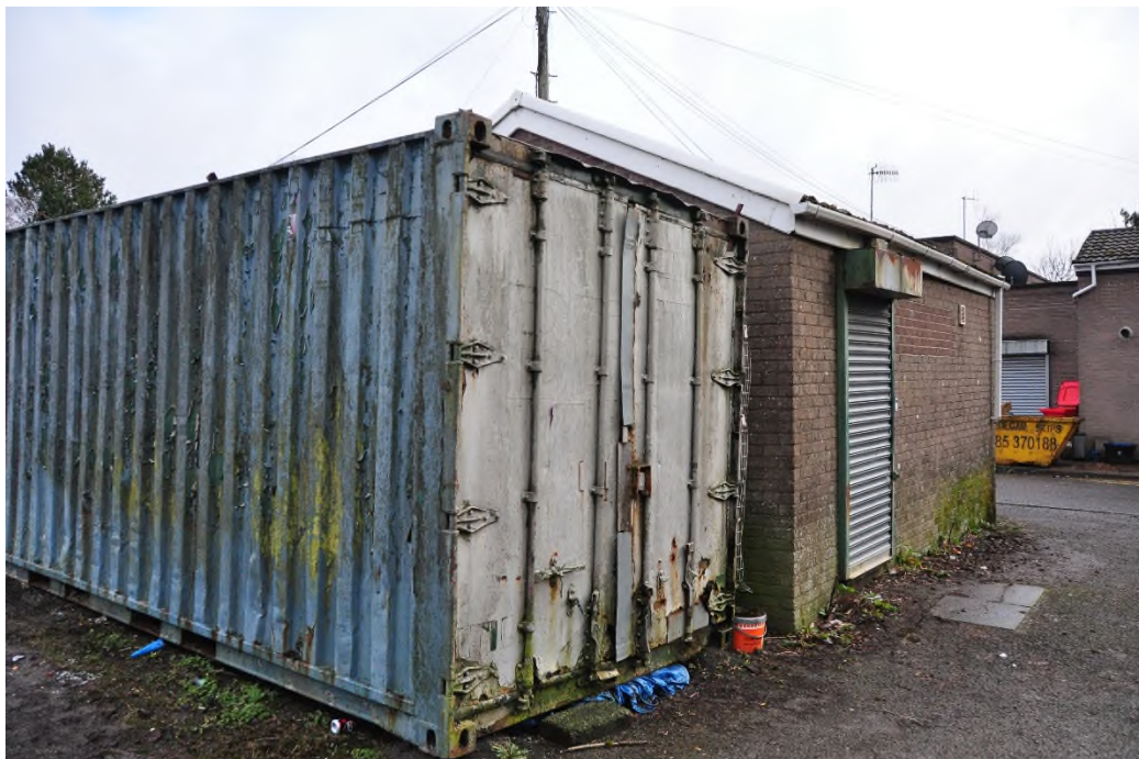
Plate 6 utility building and shipping container with negligible potential for birds or bats
