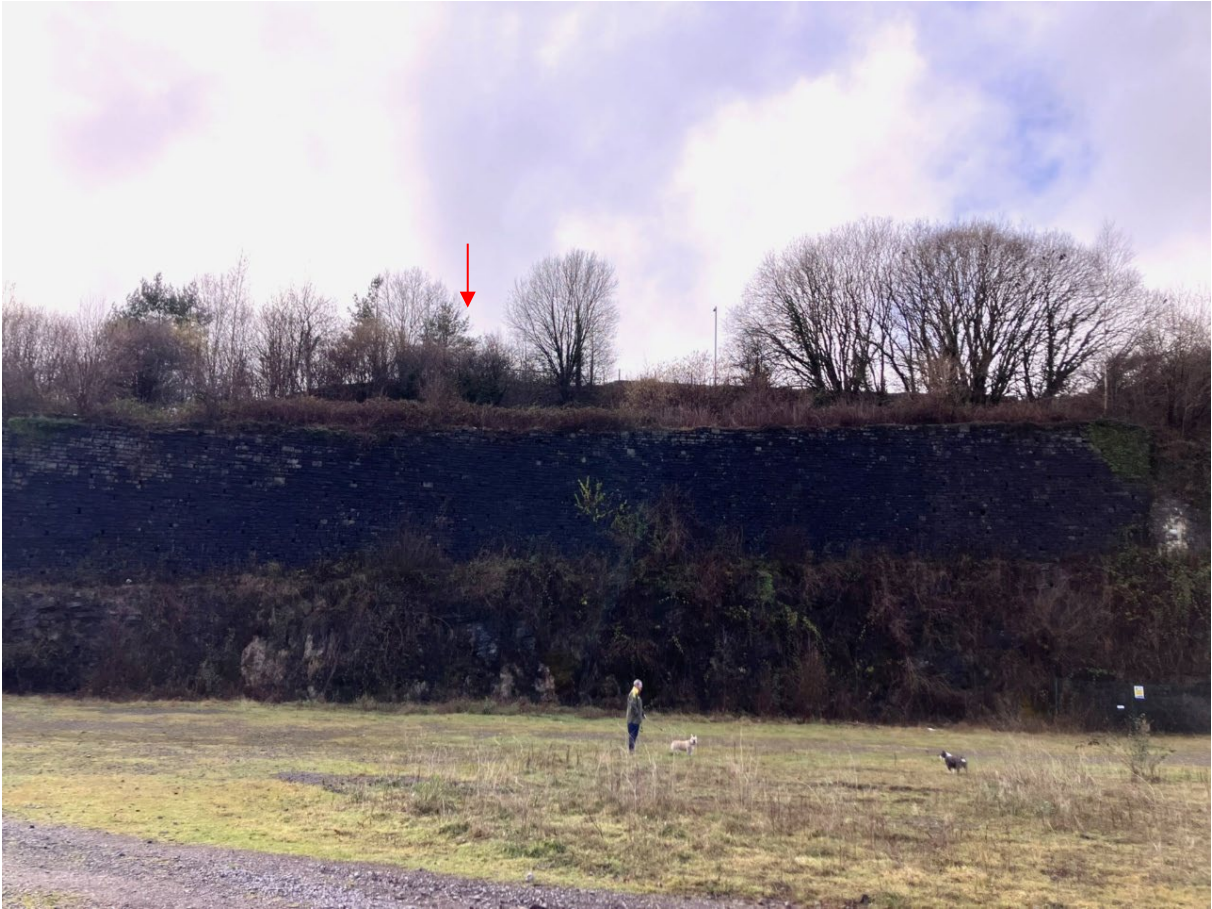
Image EDP A1.21: View south-west towards the retaining wall of the scheduled furnace bank, illustrating that the Site is visible in these views, albeit filtered by vegetation (shown by arrow).
