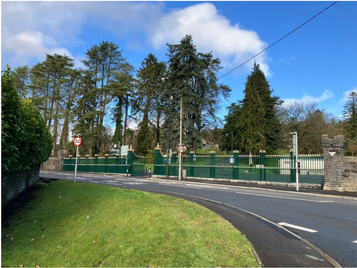
Image EDP A1.4: View north towards Cyfarthfa Park illustrating the architectural features of its entrance, comprising the Grade II listed Gate piers, Railings and Walls ( 11399 – 11402 ).
