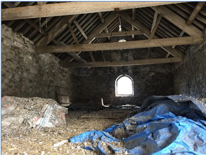
Photograph 11. Building B, western section. The first floor.
