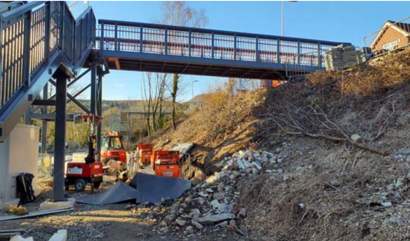
View from the bottom of the embankment south of Taff Vale, at platform level, to the towards the north west illustrating vegetation clearance
