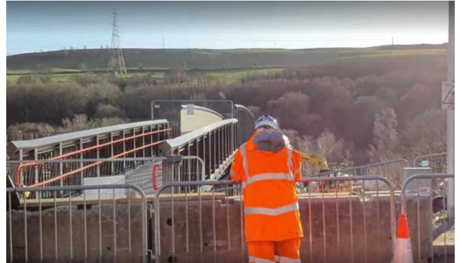
View from Taff Vale towards the south illustrating vegetation clearance and new pedestrian structure
