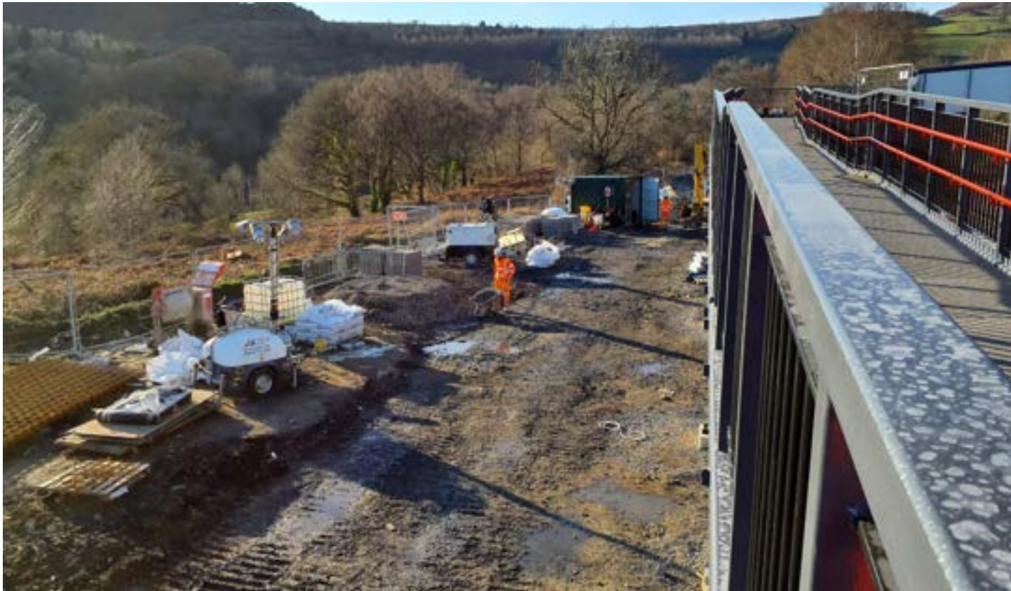
View from the ramp on the southern side of the railway tracks towards the north west illustrating existing vegetation clearance
