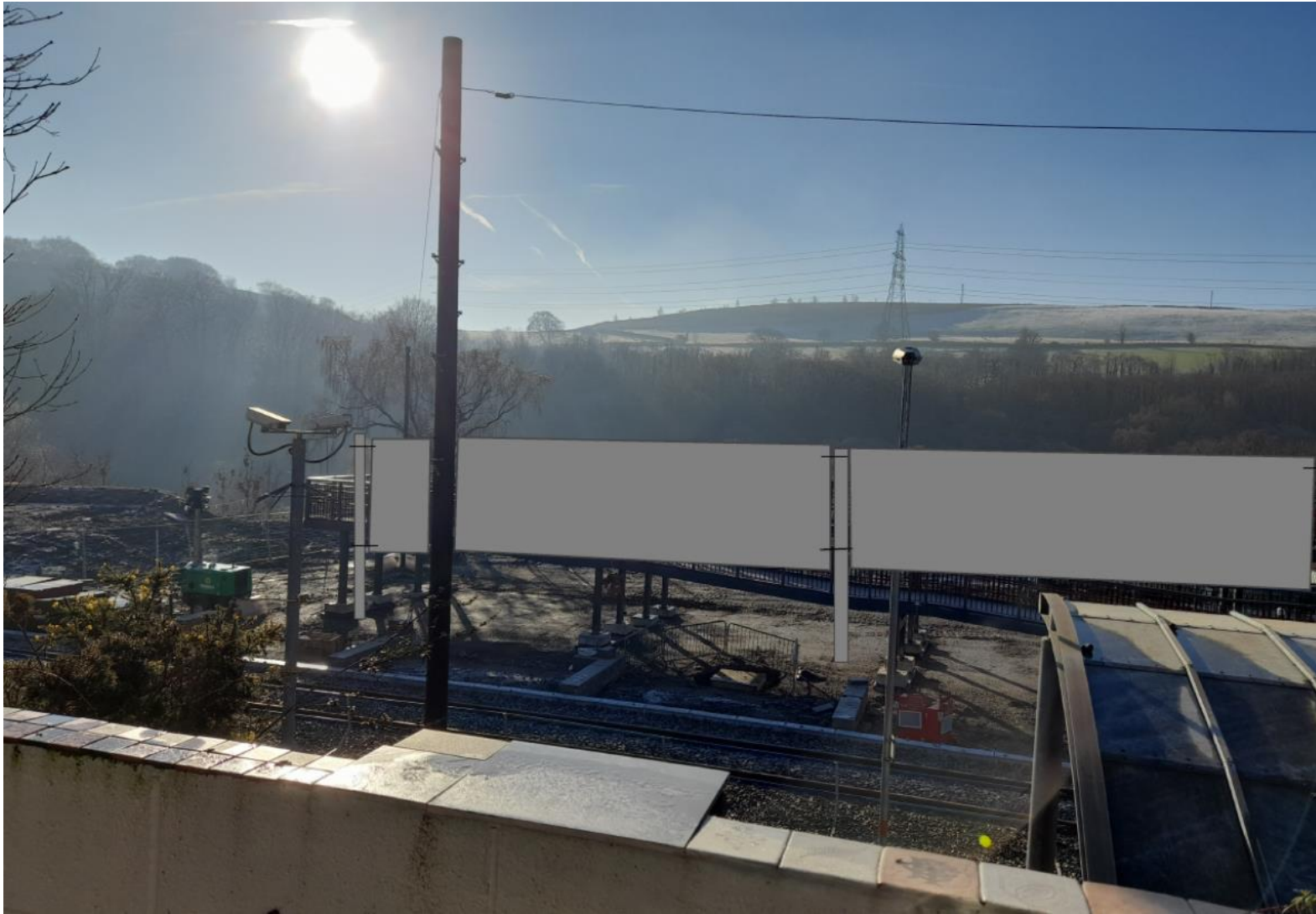
Option 2 - Independent Screen System (indicative, formed of tension wires, columns and fabric material screen)
