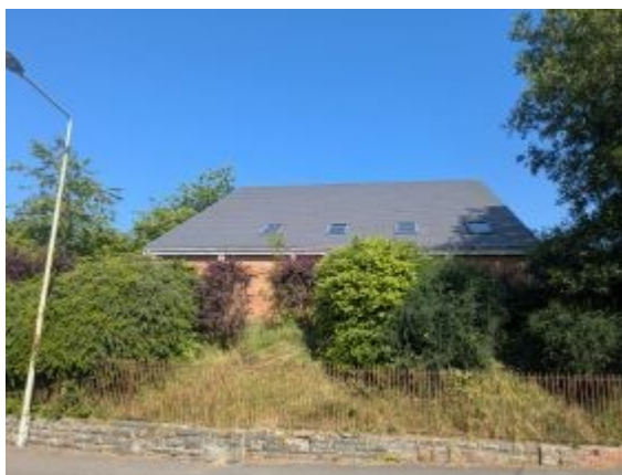
Building A (Former Church): Exterior – South-east elevation – Late 1970s, block and brick-built church with cement and trussed roof construction. Bargeboards are uPVC, the building has composite slate cement roof tiles, concrete ridge tiles and uPVC rainwater goods. The building is well maintained, and materials are in a good condition.
