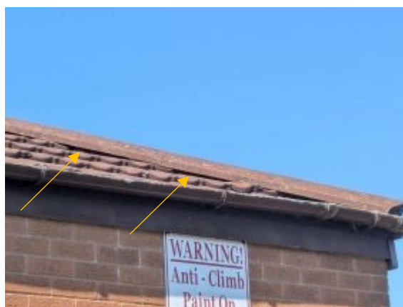
Building A (Former Church): Exterior - PRFs – Northern corner – Gap identified under hipped ridge providing a
