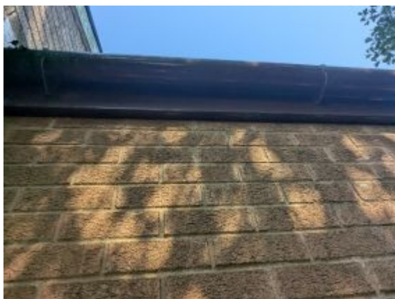
Building A (Former Church): Exterior – South-eastern elevation – Minor gaps between uPVC Bargeboards and brick surface likely too small to support occupation but bats.
