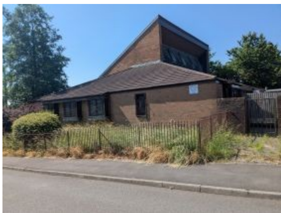
Building A (Former Church): Exterior – North-east elevation (left) and north-west elevation (right) – Late 1970s, block and brick-built church with cement and trussed roof construction. Bargeboards are uPVC, the building has cement roof and ridge tiles, and uPVC rainwater goods. The building is well maintained, and materials are in a good condition.
