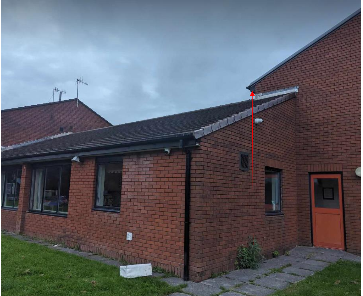
Figure 4- Location of common pipistrelle emergence point (Arrowed red)
