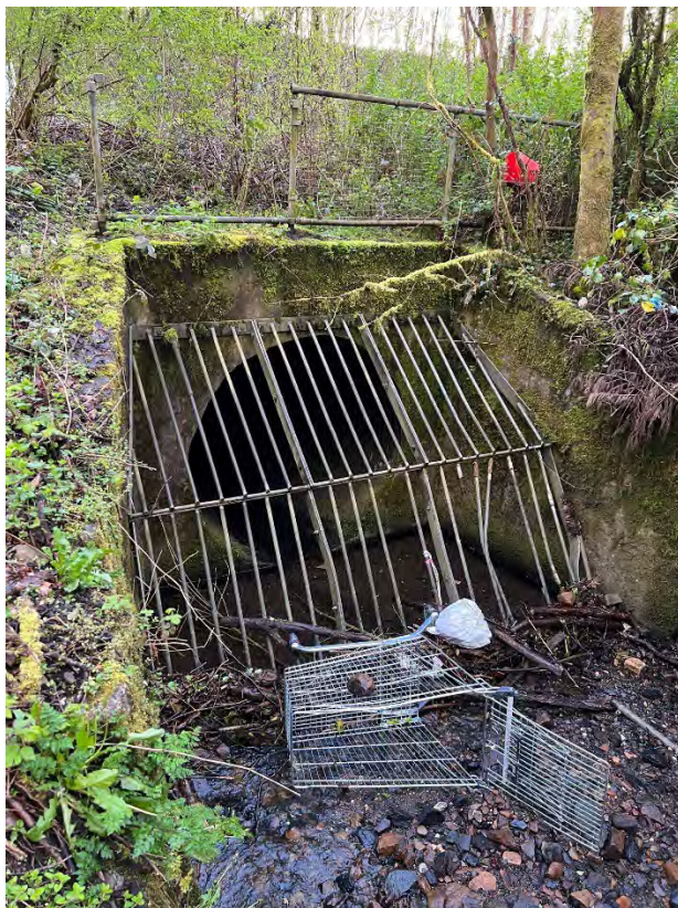
Photo 3 – Culvert taking Nant Cwm Pant Bach below A470
