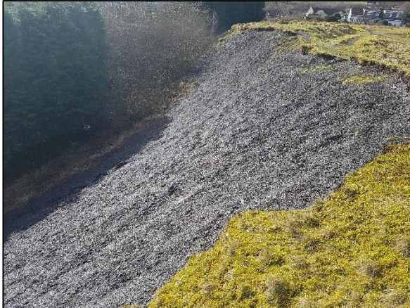
Photo 10: Exposed colliery spoil
