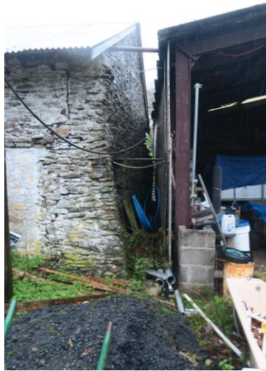
VIEW ALONG SOUTH ELEVATION: NOTE POSSIBLE FORMER WALL EXTENSION AT CORNER:
