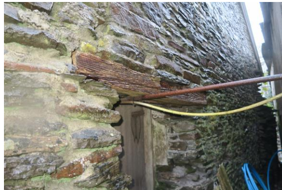
VIEW ALONG SOUTH ELEVATION: NOTE OPENING AT WEST SIDE – SECTION BOARDED OFF INSIDE:
