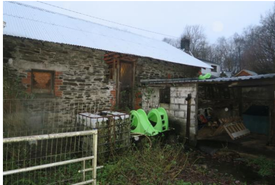
PART OF EAST ELEVATION WITH LOWER BARN:
