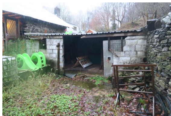
LOW LEVEL BARN:
