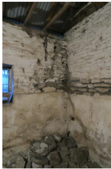
SOUTH ELEVATION INTERNAL - DETAILS: NOTE BOARDED OVER OPENING AND WITH STRAIGHT JOINTS AT CORNERS:
