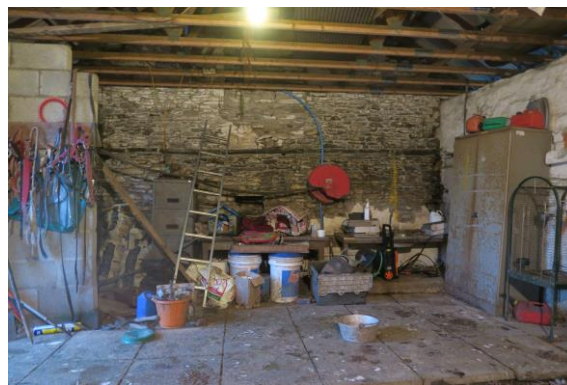
NORTH ELEVATION INTERNAL: NOTE POSSIBLE FIRE PLACE WITH STRAIGHT JOINT AT CORNER:
