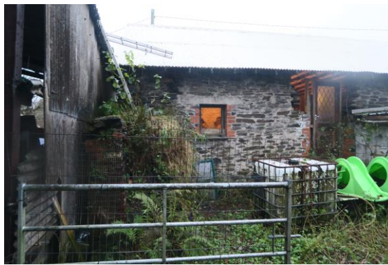
PART OF EAST ELEVATION: NOTE WALL TO SIDES OF DOOR:
