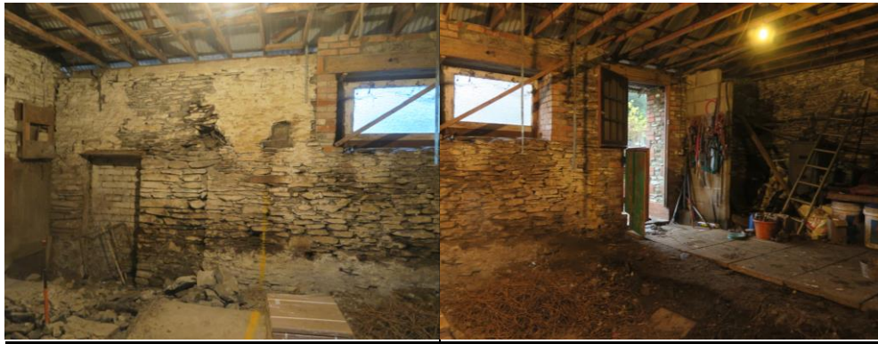
EAST ELEVATION INTERNAL: NOTE INFILLED OPENINGS WITH STRAIGHT JOINT AND STRAIGHT JOINT AT CORNER:
