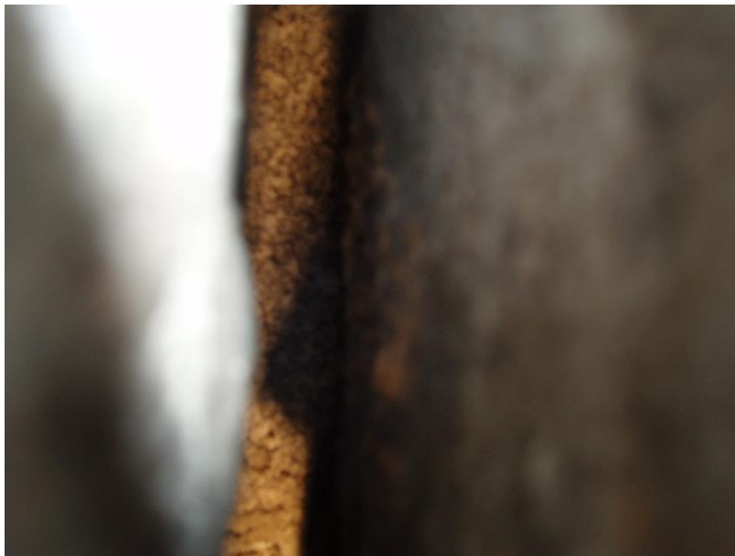
Looking into the main crack with the endoscope, no evidence of bats
