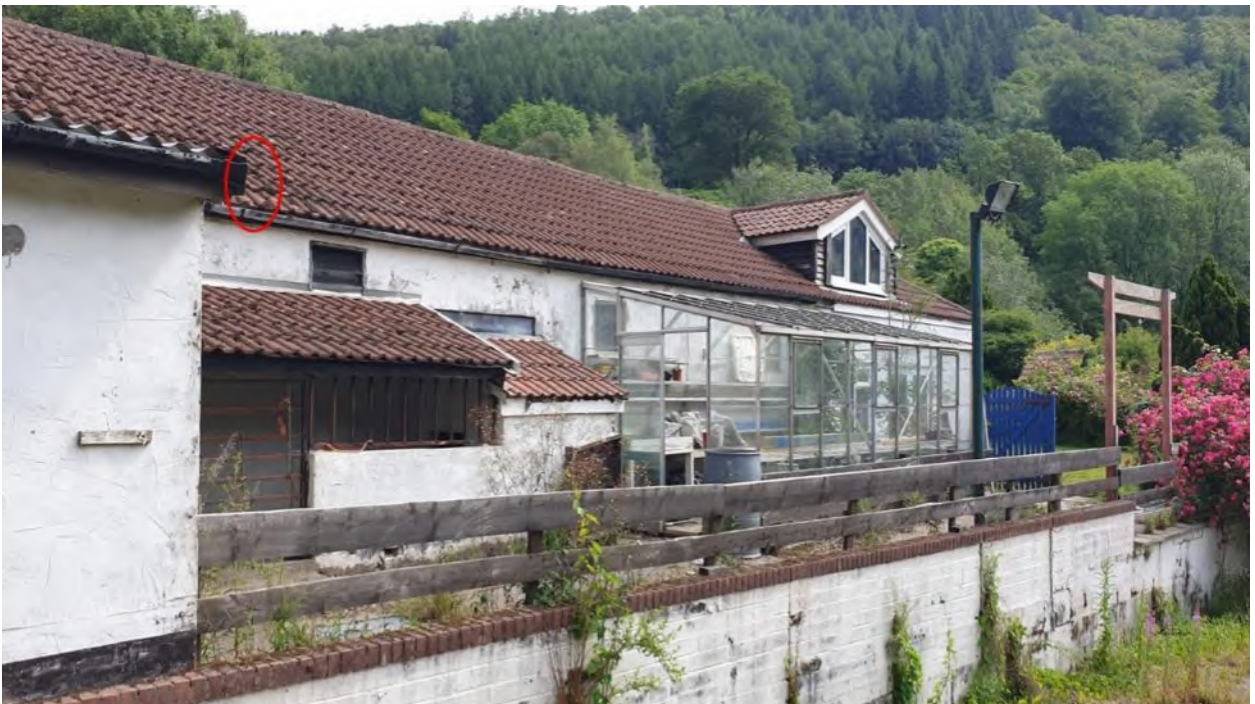
4) Bat emergence point on south elevation
