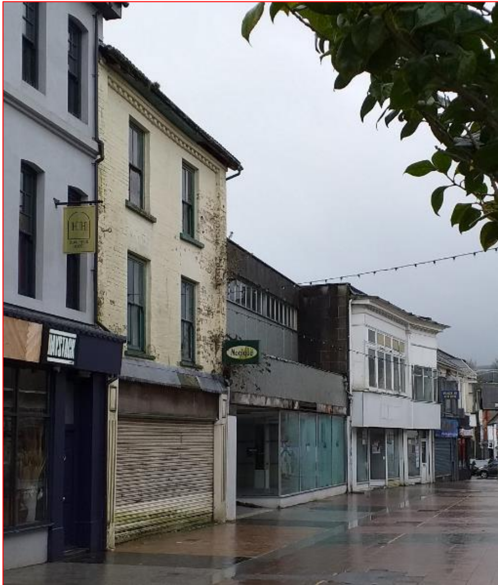
Plate 1 – Principal front (west) elevations to nos. 34-38 High Street. Note that this view is taken from the north looking south-east.
