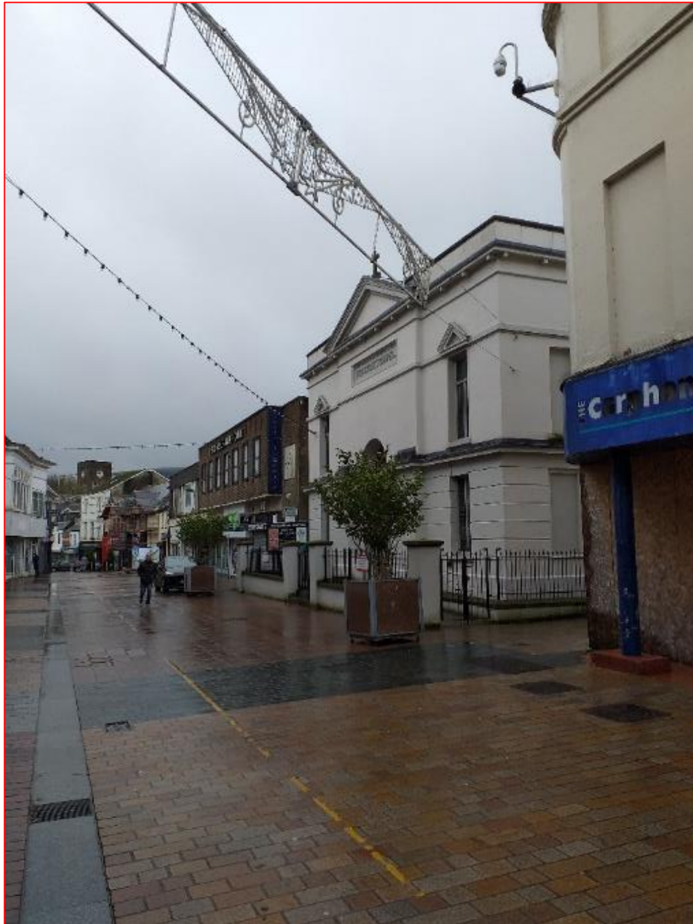
Plate 12: Grade II listed High Street Baptist Church (Cadw 11451) taken from High Street, facing south-west and showing its position on High Street.
