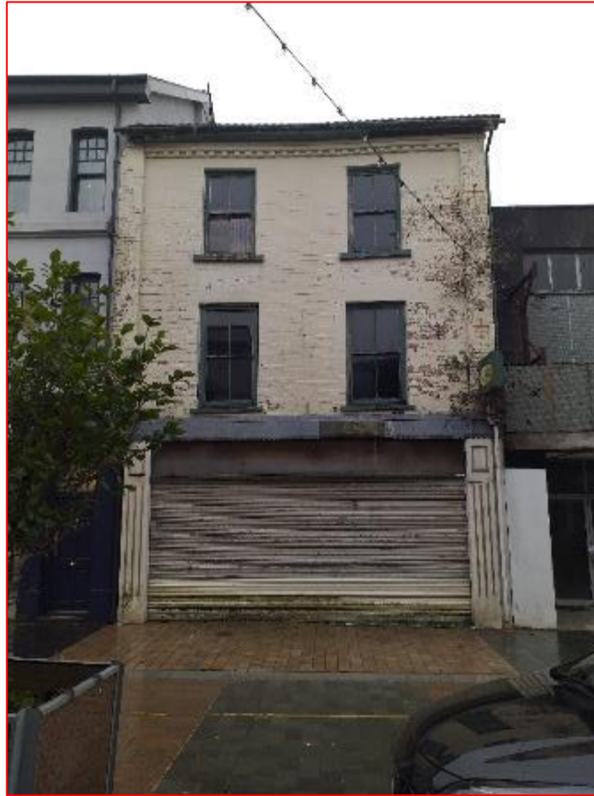
Plate 2: Principal west elevation to Monique's Building, located at no. 38 High Street
