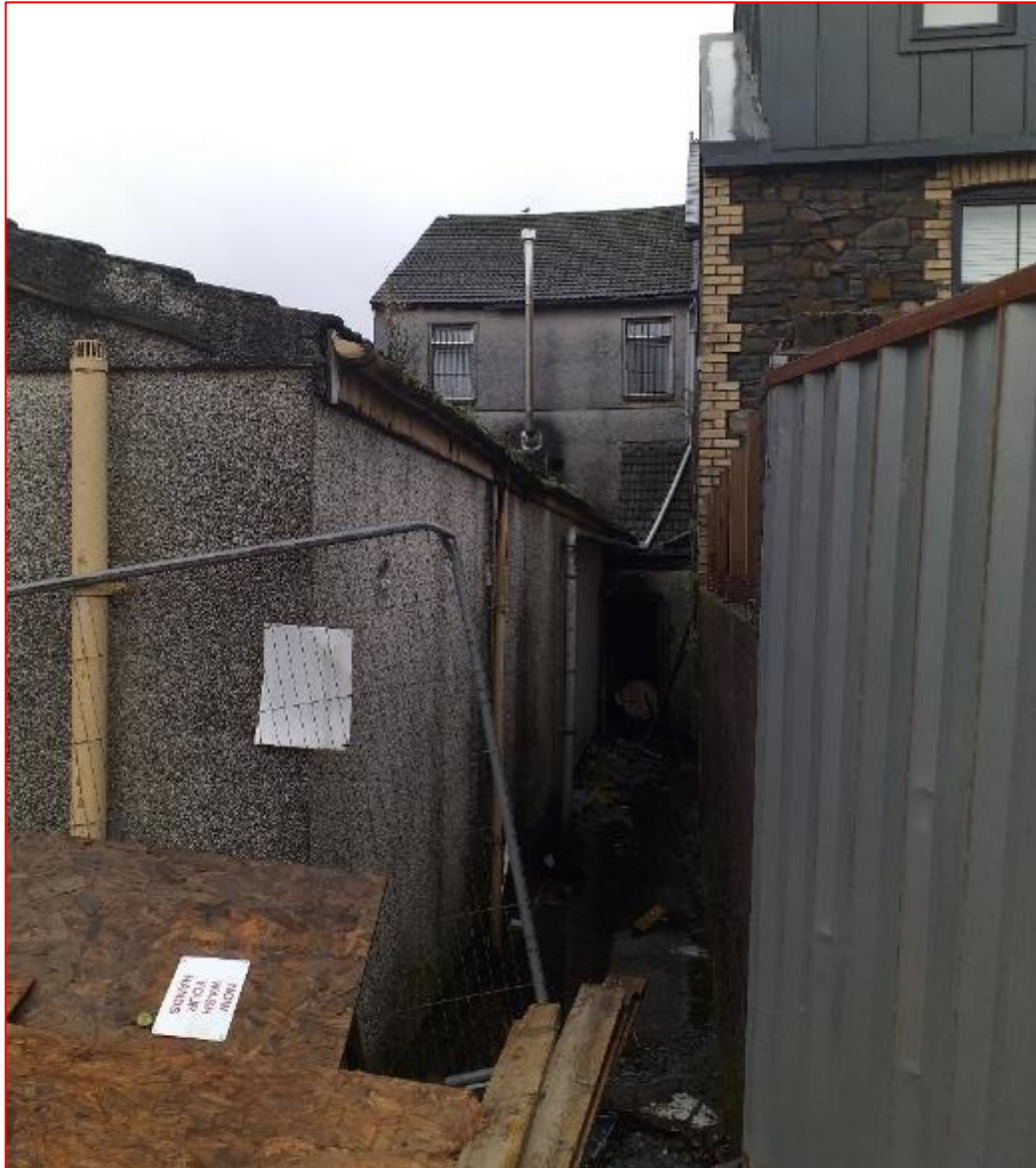
Plate 7: Rear elevation of Monique's Building at no. 38 High Street. Note the narrow back passage.
