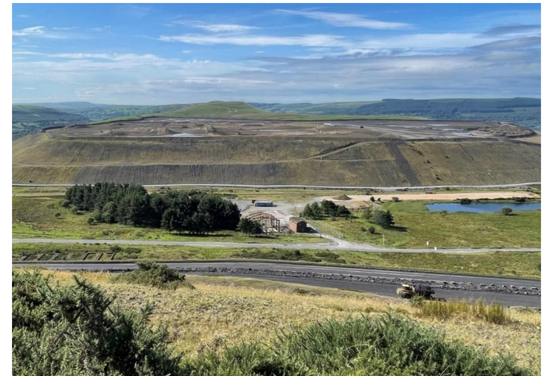
View of overburden mound OB3 that will remain as part of the final restoration scheme
