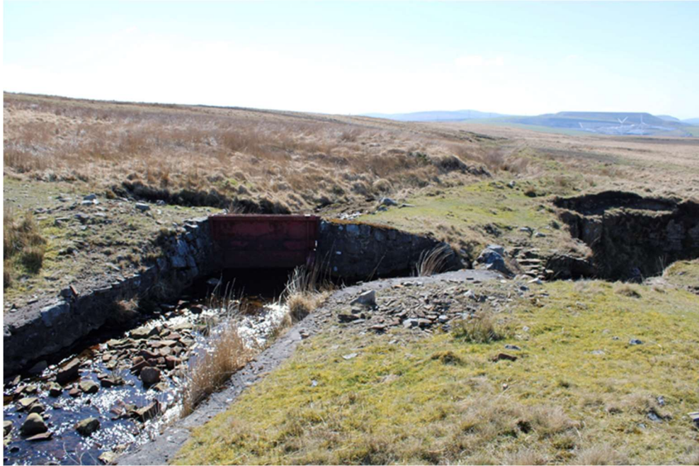
Photo 13: Section of Nant Morlais within revetted banks close to Pitwellt Pond
