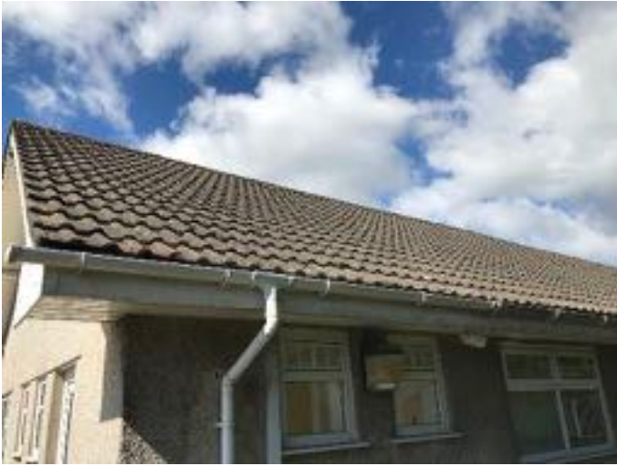
Example view of roof line
