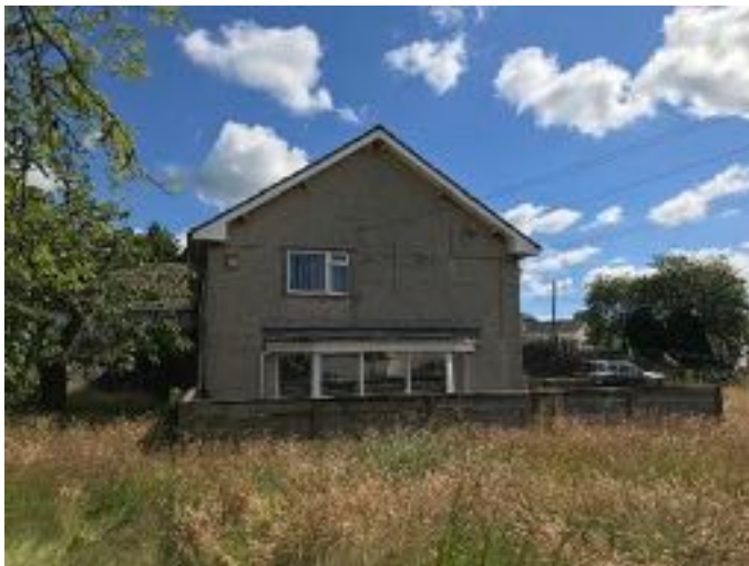
South gable end of building
