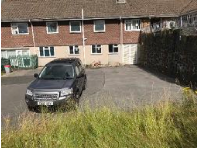
Tarmac hardstanding to east of building
