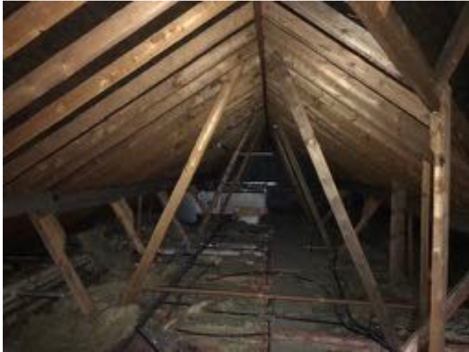
View of internal attic space
