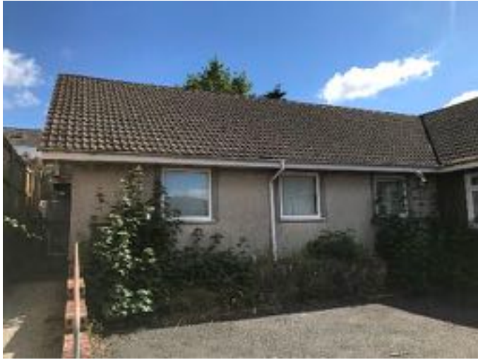
Example view of roof line
