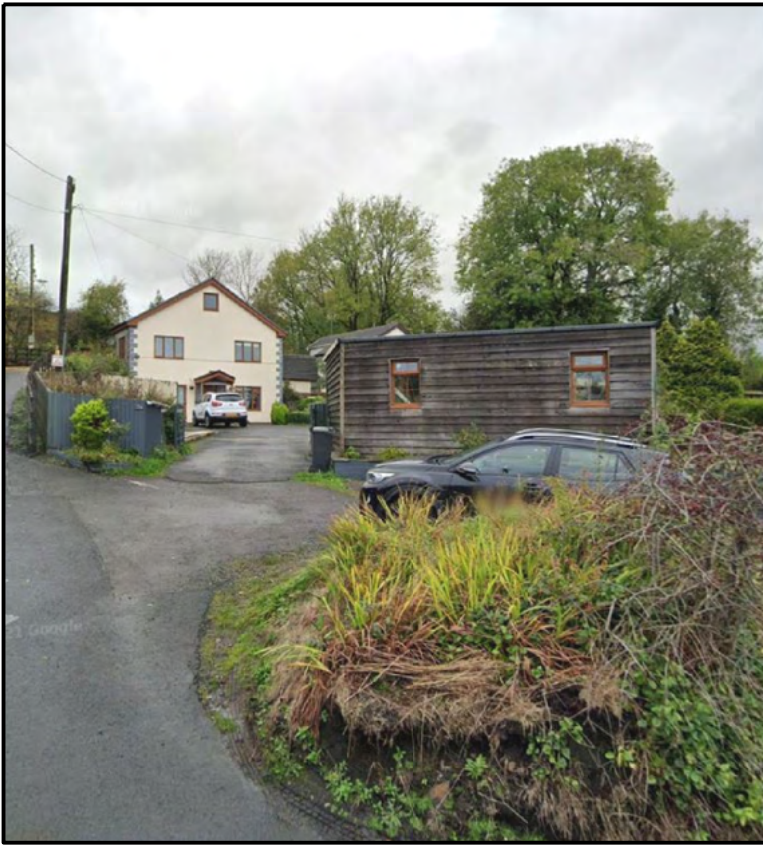
Photograph of Existing Property from Main Road
