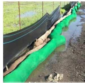
Fig.3.7 – Silt fence
