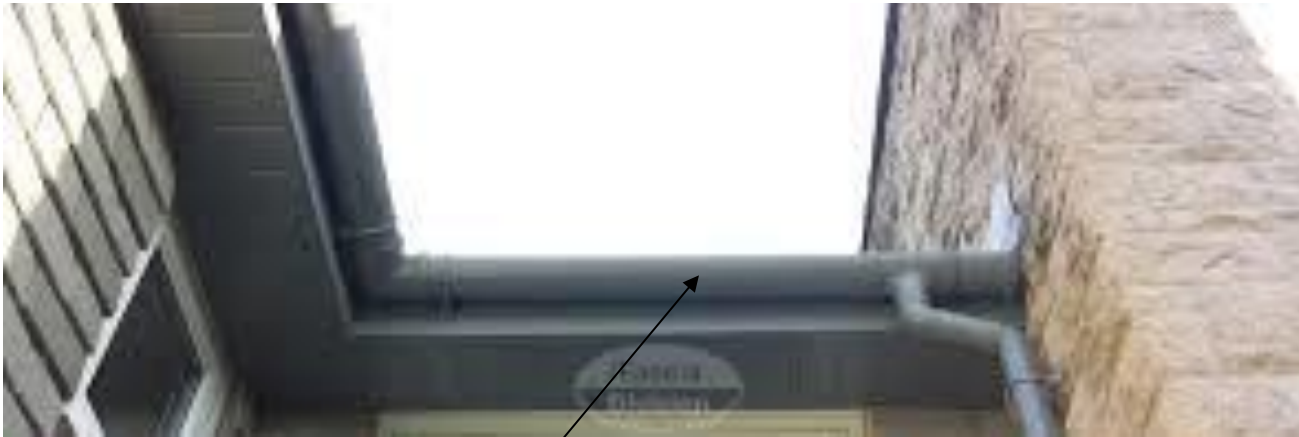
Gutters and downpipes
