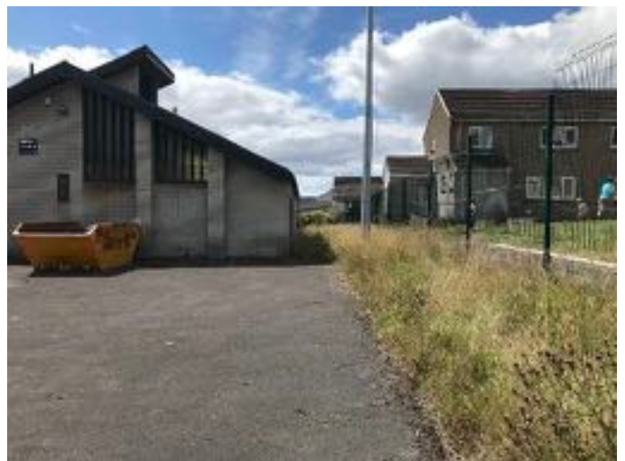
North boundary of site looking west
