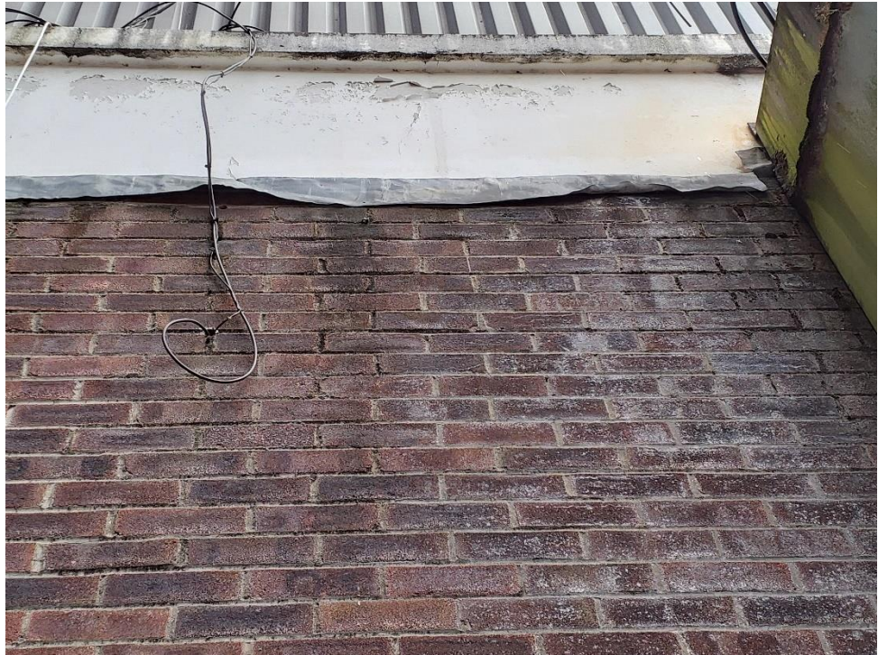
Photo 11: Lifting in lead flashing creating gaps (B3).
