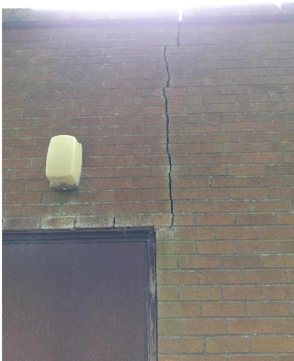
Photo 14: Crack in brickwork of the old water pumping station building (B7) to the east.
