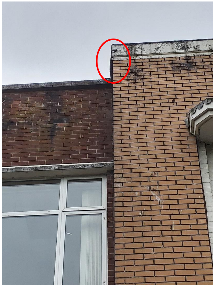
Photo 8: Lifting in roof felt creating a gap (B1).
