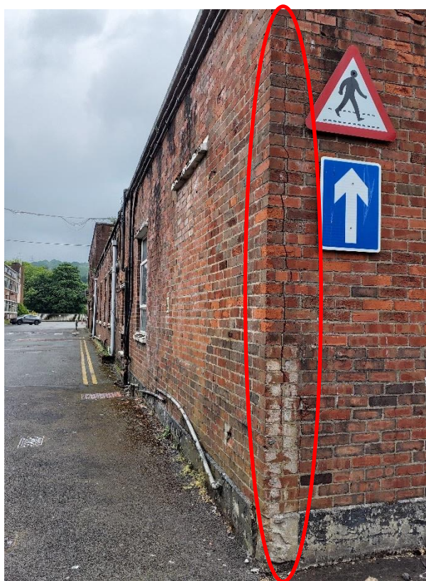
Photo 13: Crack in brickwork of smaller brick building (B6) to the south of the main Hoover site.
