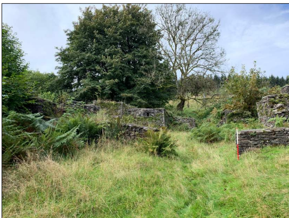
Plate 34. West facing view of Pen-y-lan Farm.
