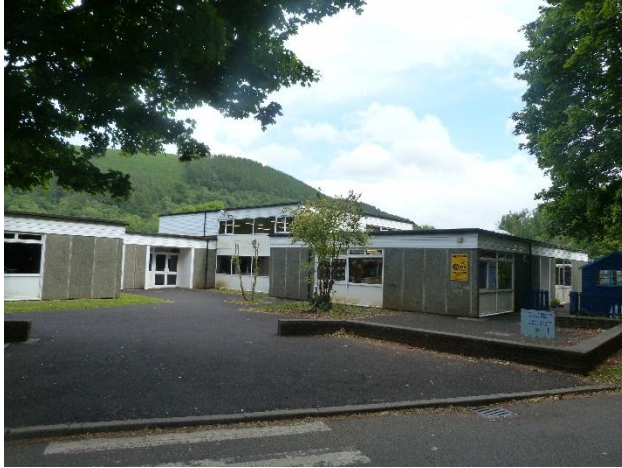
Photo 7: Western aspect of B1, looking south-east
