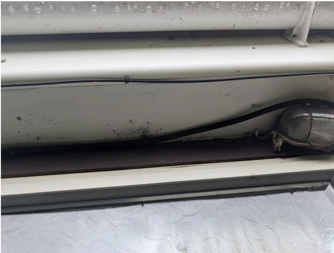
Plate 2- close up of sealed eaves
