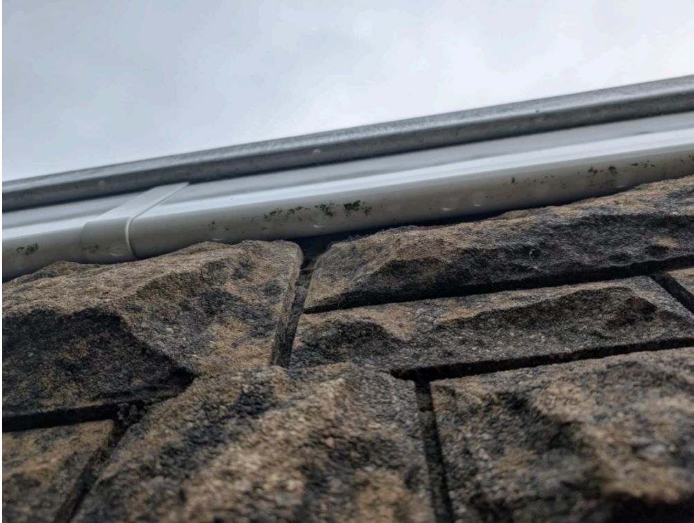
Plate 5- example of small gap beneath fascia on side elevation
