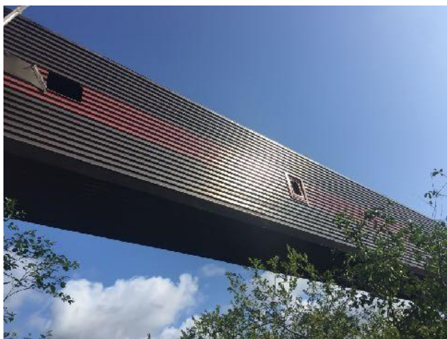
View of gantry over River Taff
