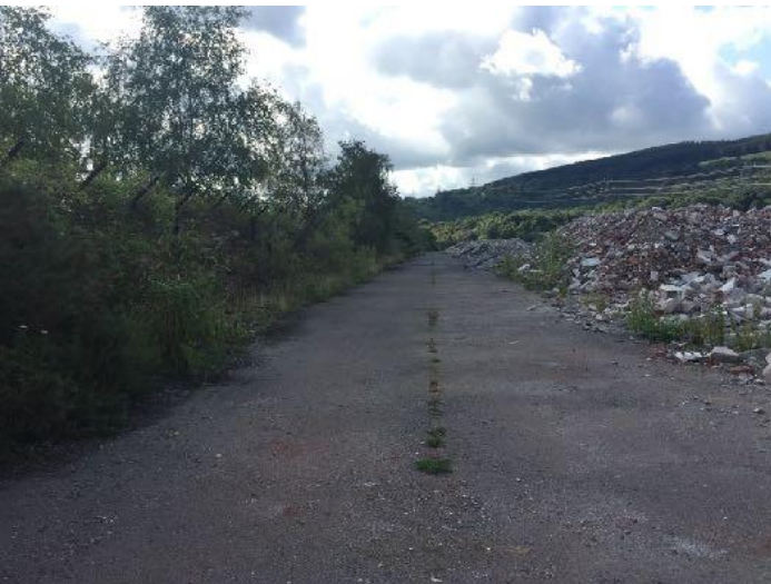
Tarmac road along north east looking south
