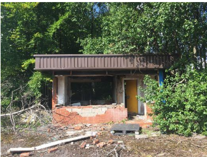
Remaining small building
