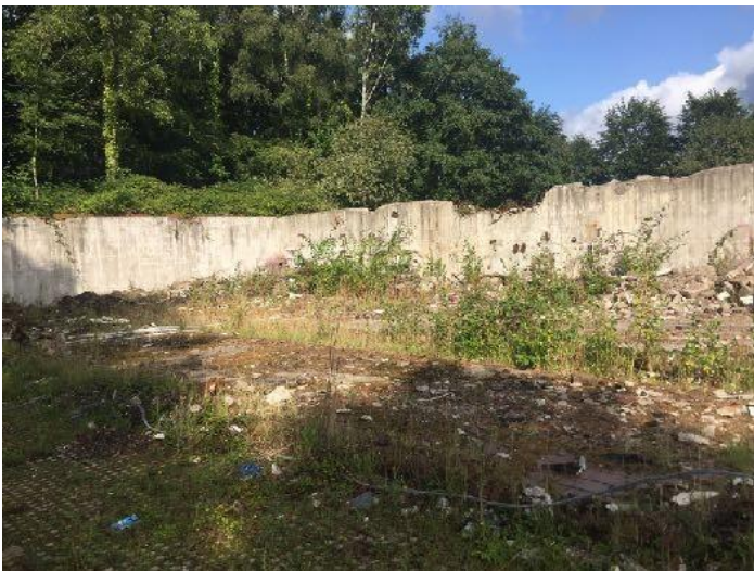
View of building foundations
