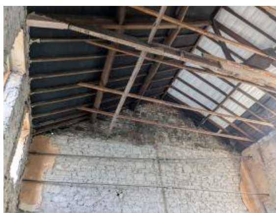
PRF – Internal, upper-floors. Bitumen membrane.
