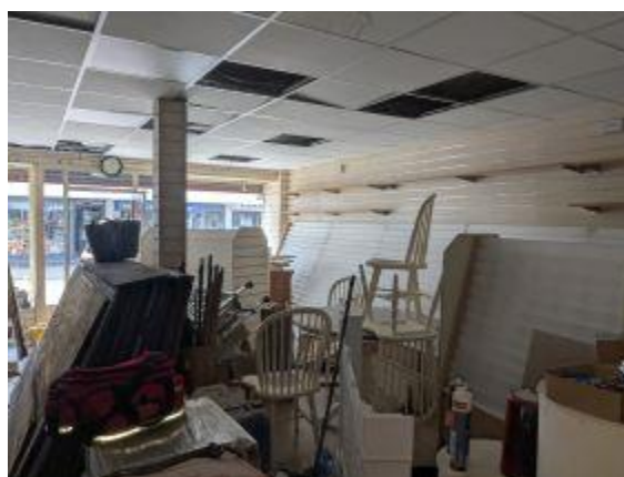
Lower floor – utilised as storage.
