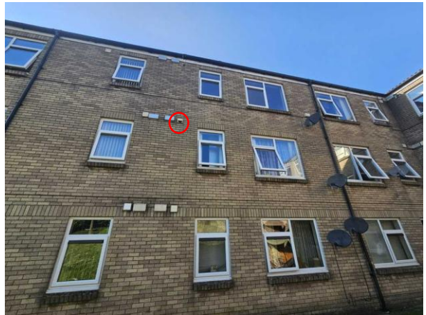
Photo 6: Missing mortar on western gable
