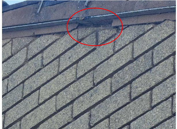
Photo 6: Missing mortar on western gable
