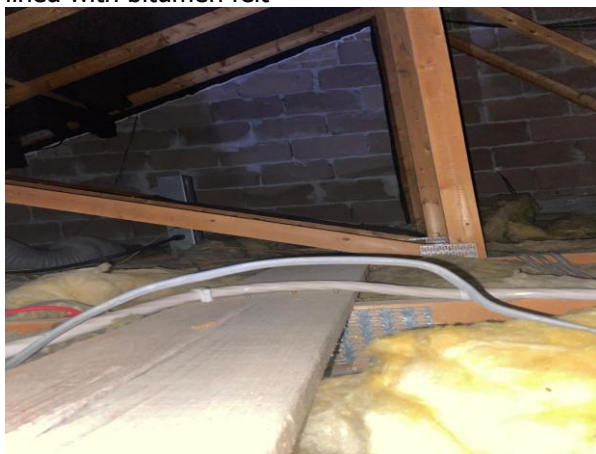
Photo 13: Internal loft space on eastern elevation, lined with bitumen felt
