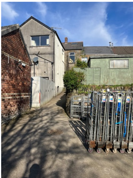
Plate 8: Bat and bird boxes can be affixed to the area of rendered wall below the eaves.
