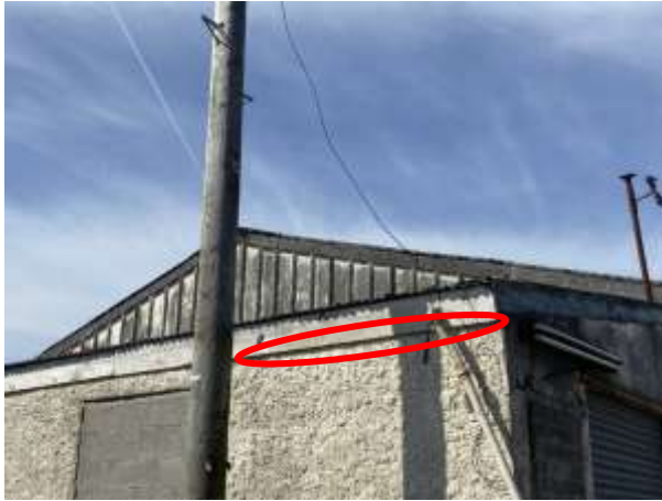
Photo 9: Cavity in External Wall Northern Front
