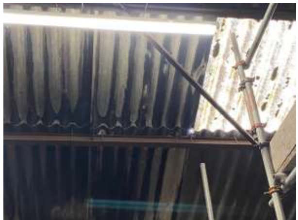
Photo 6: Overlapping Corrugated Sheets
