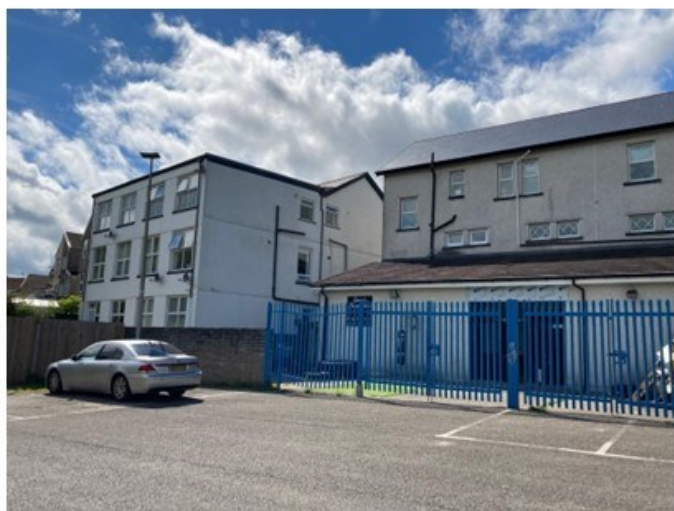
View of rear of Properties on Perrott Street from Car Park
