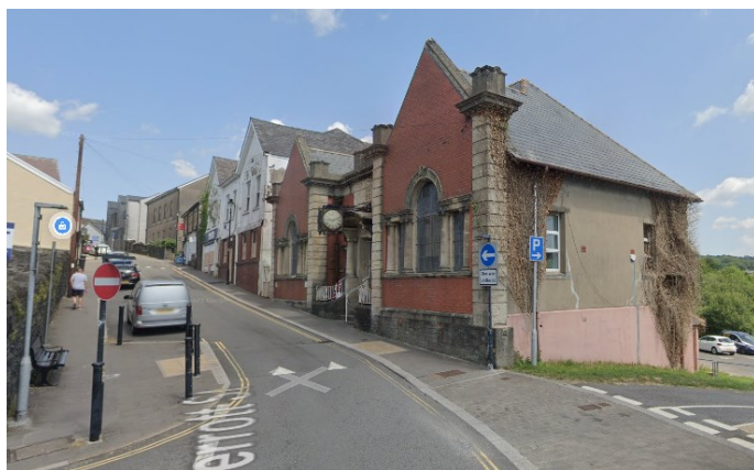
Gable Frontages along Perrott Street
