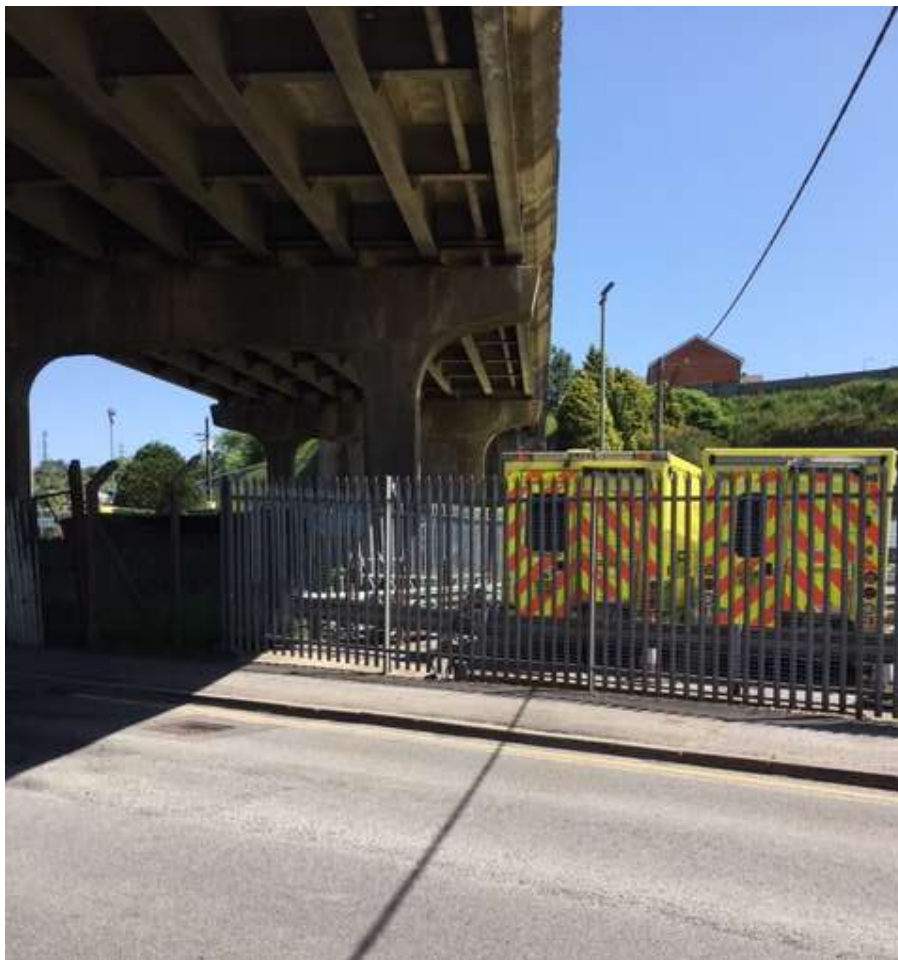
20. View under A465 eastward toward MMA site, elevated housing of Wern Street visible in background
