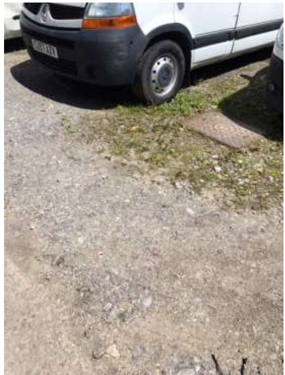
6. Hard surfacing to Site H
