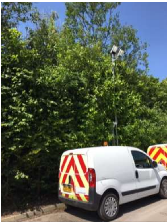
3. Site H – Lighting column to western boundary
