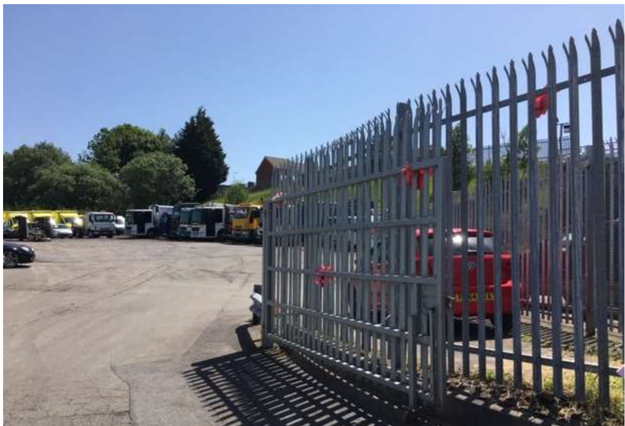
13. Steel Palisade fencing and gate to main customer access to MMA site
