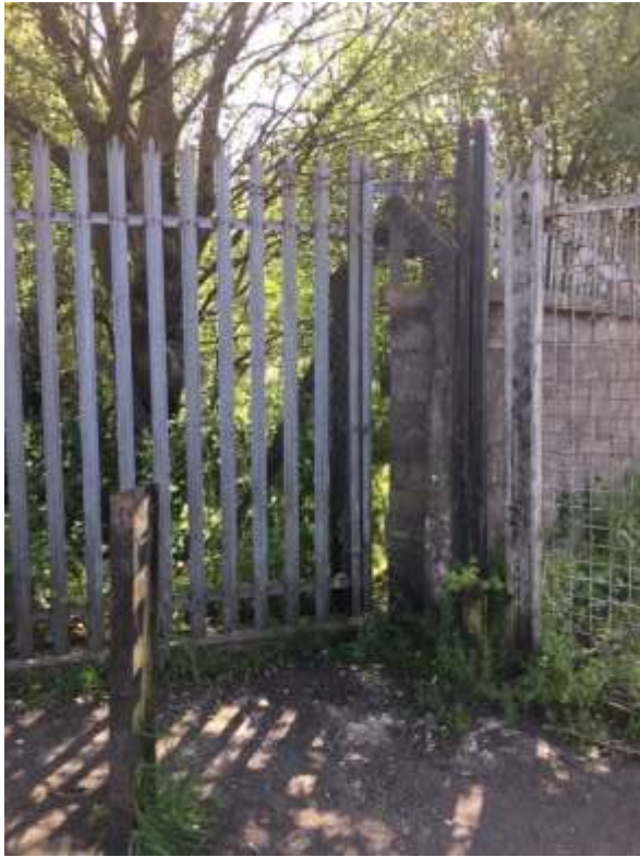
1. Looking in to pathway from bottom of site H
