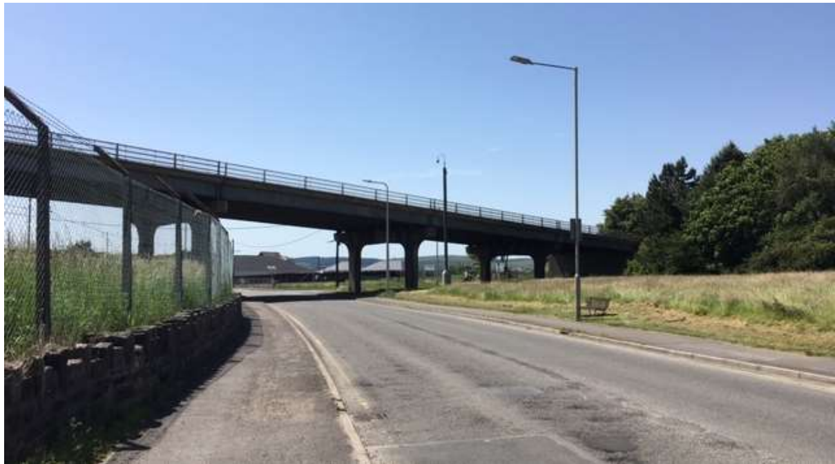
16. Pant Road running beneath A465. MMA site and security fencing visible to left
