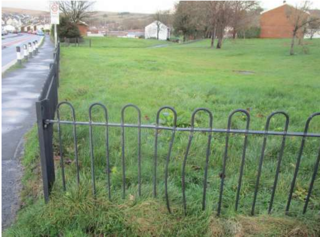
21. Utility covers in Hafod land
